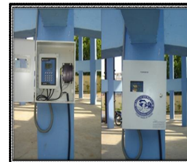
Fig. 9 Installation of flow meter
